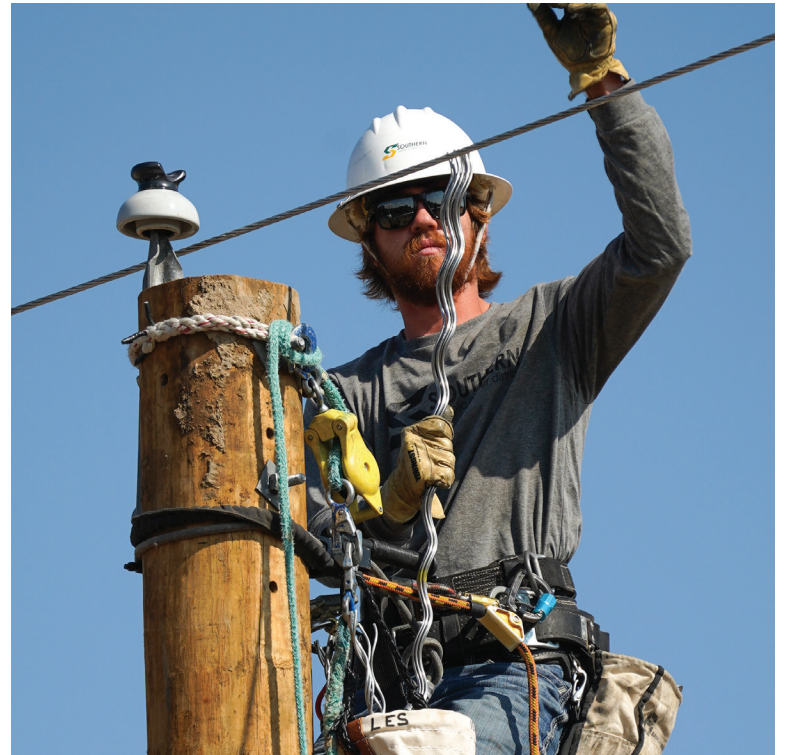
Above: Cole Sundberg installing armor rod on the primary conductor in the Armor Rod event. - Photo Courtesy of Lincoln Electrical Systems
