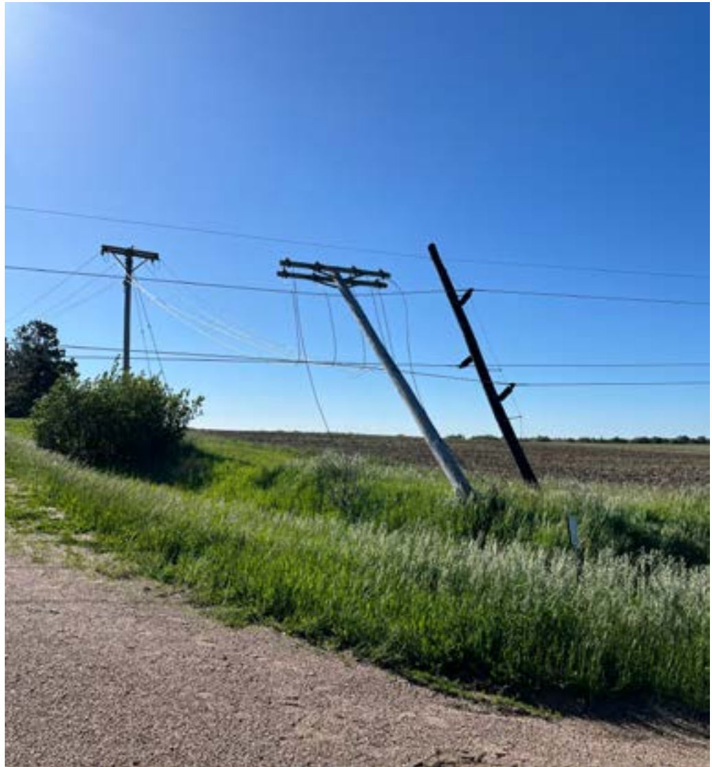
Above: May storms knocked down sub-transmission and distribution lines in the Central City area. - Photo by Todd Barger
